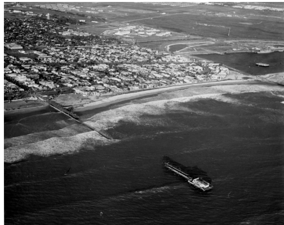
The washed out Seal Beach pier following the storms of the 1983 El Niño. Image from Michael Dobkins.
