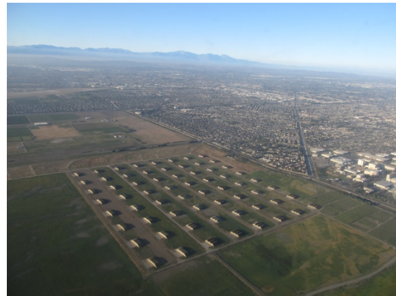
The Naval Weapons Station is a potential source of hazardous material releases. Image from Ken Lund.
